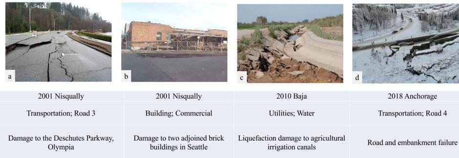
**Figure 3:** Examples of damaging liquefaction occurrences across three US events. First row indicates year and location of event, second row indicates category and subcategory of each damage, and third row gives a brief description of the damage shown. Pictures and text obtained from GEER Association reconnaissance reports for each event.
